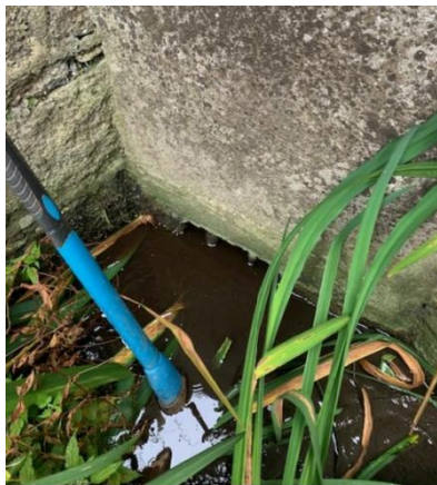
Photos 1.2 and 1.3: Grated Drainage Openings Along the Eastern Boundary
