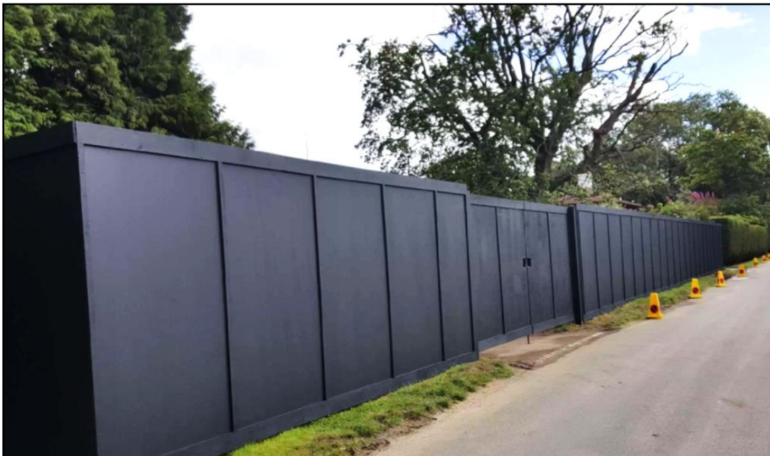
Photo 9.1 – Typical Site Hoarding Arrangement
