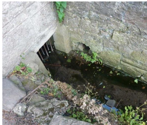
Photos 1.2 and 1.3: Grated Drainage Openings Along the Eastern Boundary
